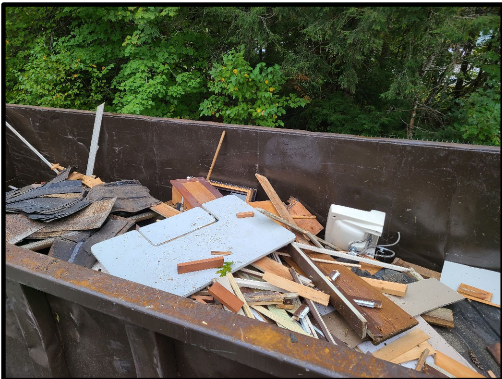
Photo 16: Construction and Demo Debris Roll-off
