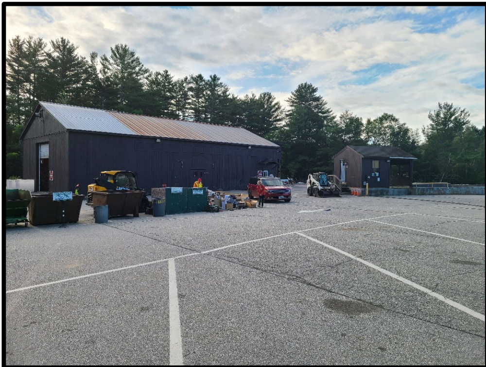
Photo 32: Swap Shop Area – Looking Southeast
