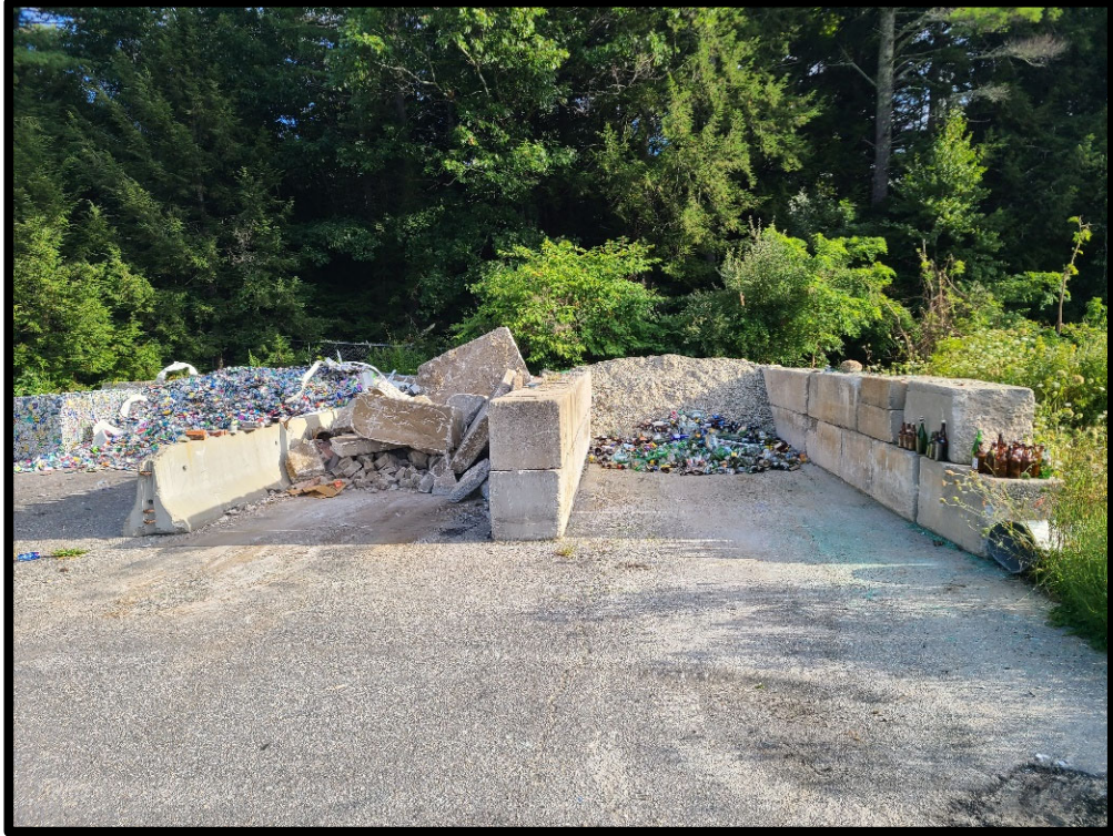
Photo 29: Recycling Bunker Area – Looking North
