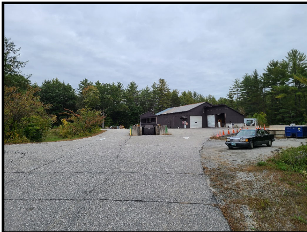
Photo 2: Site Entrance – Looking North
