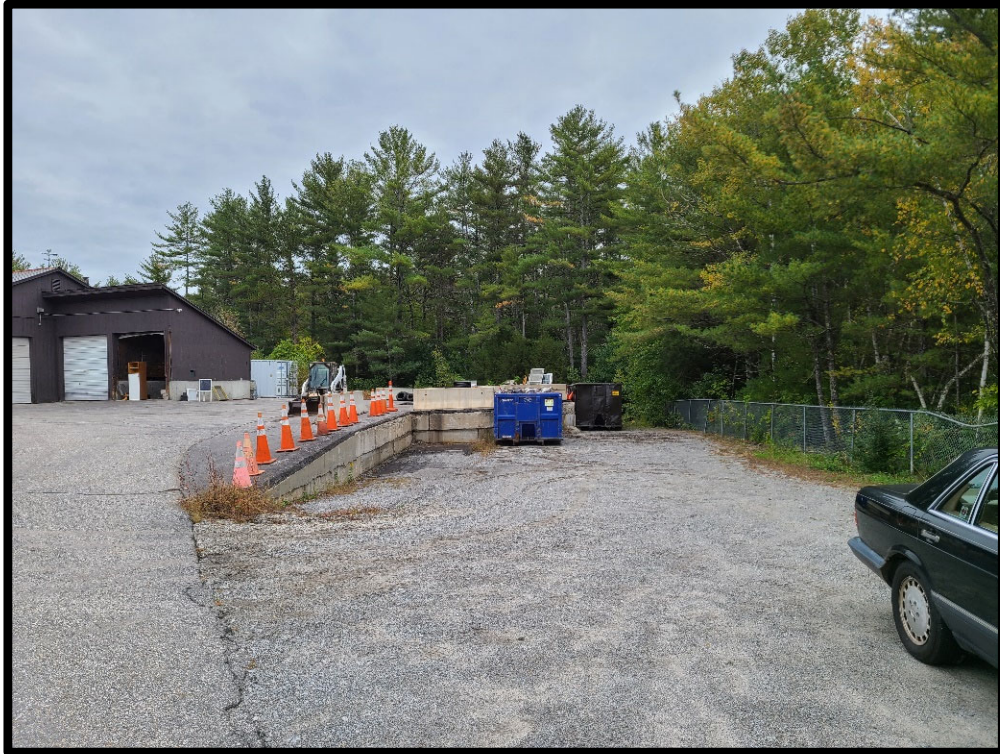
Photo 15: Metals & C&D Roll-off Container Wall – Looking East
