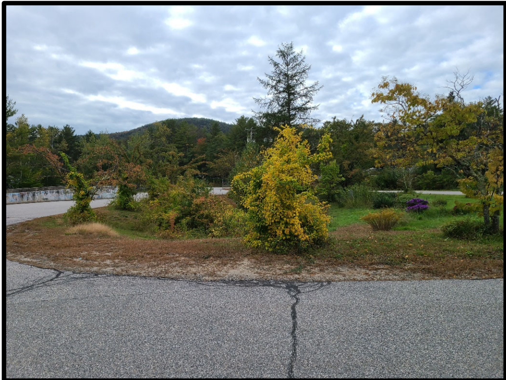
Photo 30: Transfer Station Island/Pond Area
