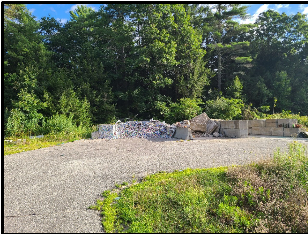
Photo 28: Recycling Bunker Area – Looking North
