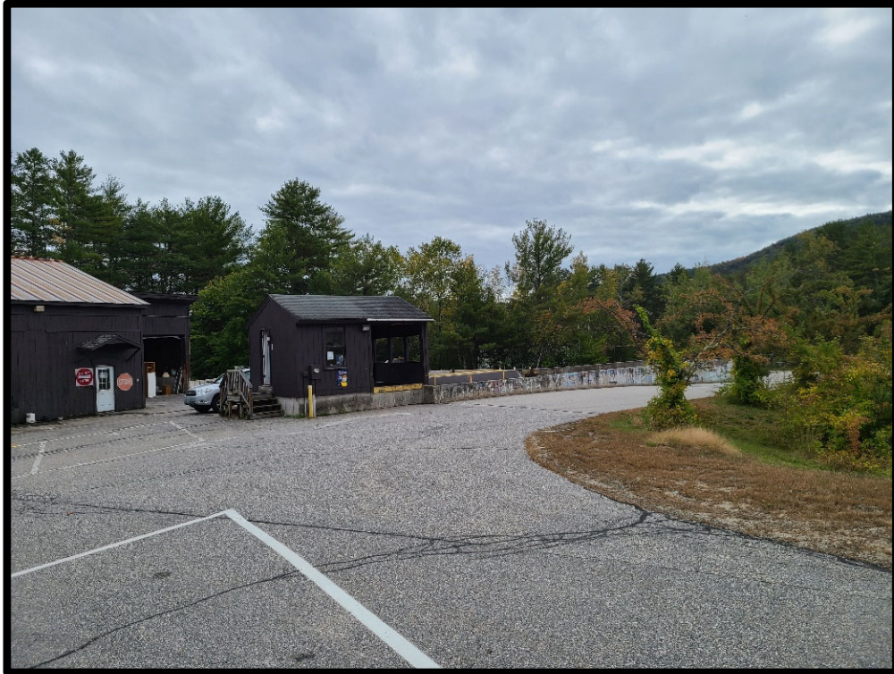
Photo 3: Office and MSW Hopper – Looking Southeast
