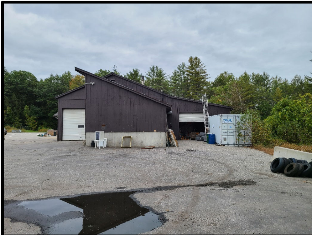
Photo 20: South Recycling Building Elevation – Looking North
