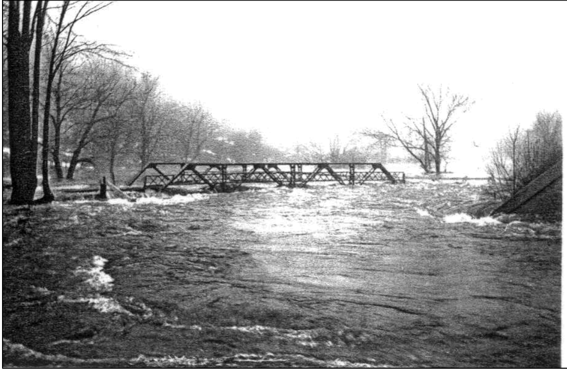
Warner River at Roby Road Bridge
