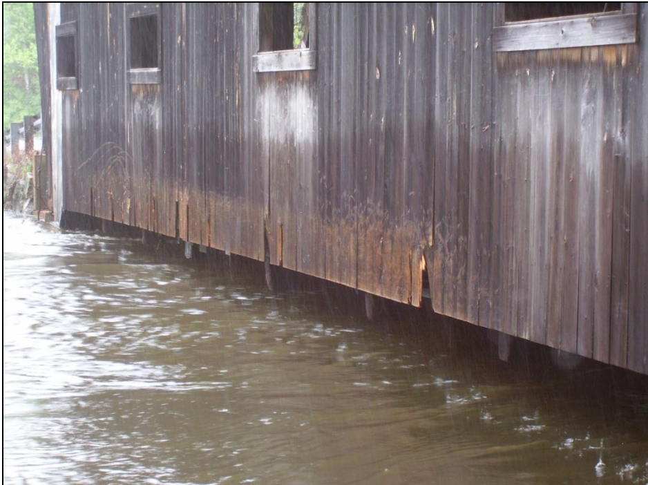
Joppa Covered Bridge over Warner River
