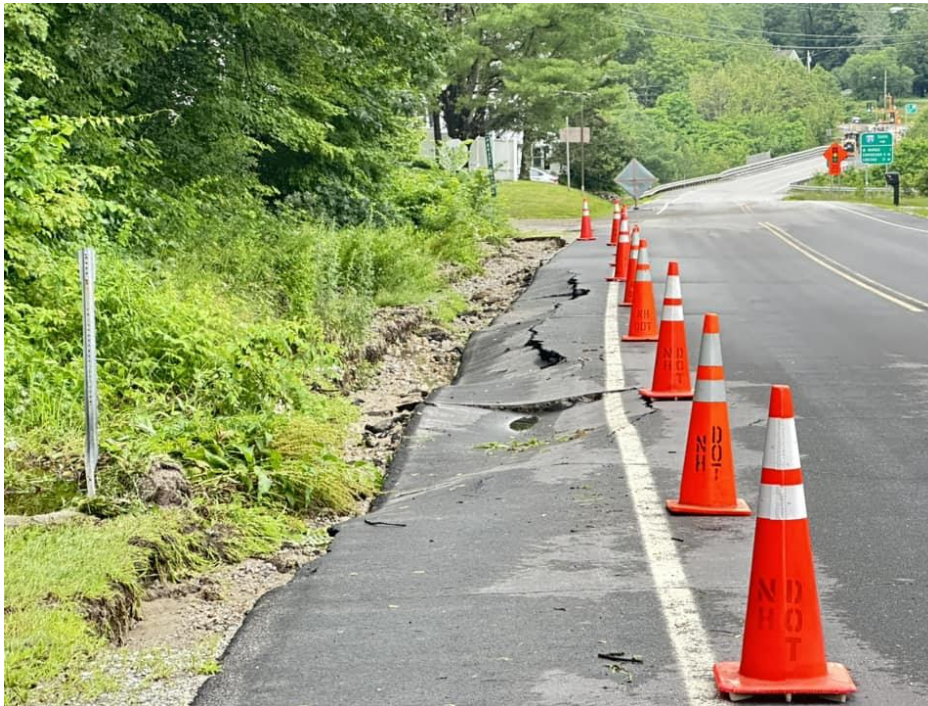
Flooding causes major road drainage damage on NH-103, near Exit 8
