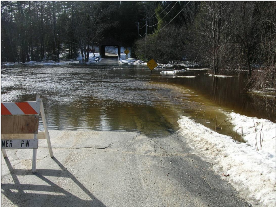
Facing the Dalton Covered Bridge on West Joppa Road, January 2018
