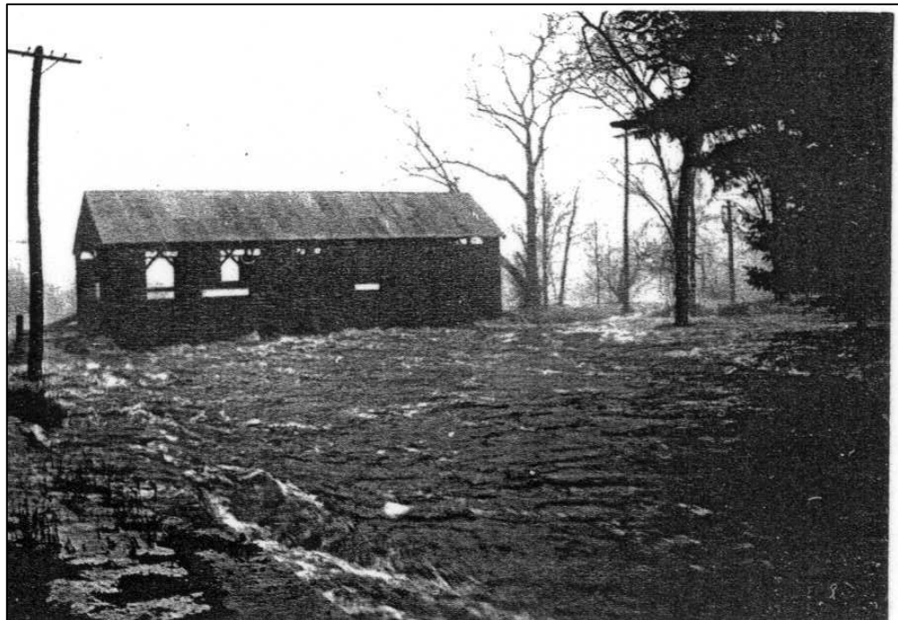
Warner River at Covered Bridge
