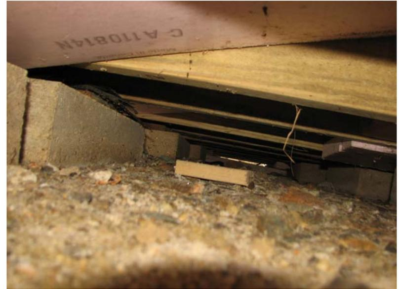
Rigid board has been stuffed under the floor with minimal impact. As heat will conduct to cold thorough thermal bridging and gaps. The good intentions behind “Every little bit helps” is lost on thermodynamics.
