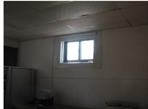
The above pattern suggests water leakage – probably in the past – and perhaps before exterior patching below the window. Gutting this area of wall to make sure all has effectively dried is advised for building durability and health benefits.
