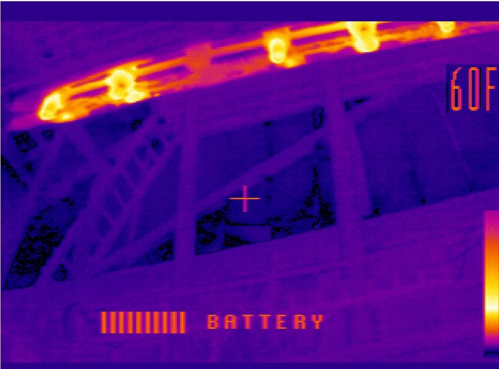
Gut plaster, remove fiberglass, dense pack, and install rigid for a continuous and effective barrier to reduce heat loss and make all those pretty colors go away!
