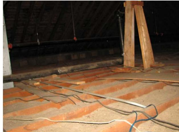
With no access to the ceiling under this roof and no drawings, the insulation is an unknown. However, Ed believes he saw an 1" rigid foam, so for estimating purposes, the roof is assessed at R5. The next step would be to make a hole in the ceiling and do a physical inspection of this assembly.
