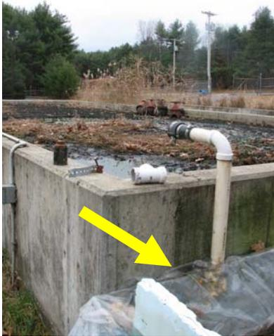
This line has been insulated but also uses a heat tape to prevent freezing – especially where it enters the reed beds where it is most unprotected.
